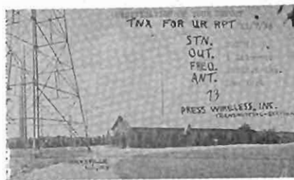
A telegraph station that broadcasts, and a commercial station that verifies, is the unusual record of W9XDH the Press Wireless station at Elgin, Ill. This card shows the transmitting buildings of another Press Wireless station, W2XGB, at Hicksville, N. Y. (Courtesy of A. D. Jordan).
